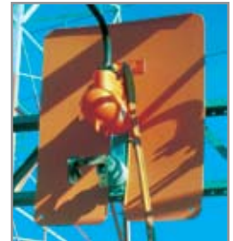
Barrier and Switch Jaw Guard installed on a Substation Switch.
