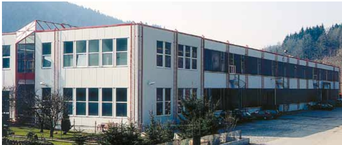
Main manufacturing facility on corporate complex.
