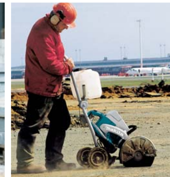
Precision cutting in asphalt with the disc cutter mounted on the saw cart.
