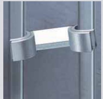
Completed sheet connection
