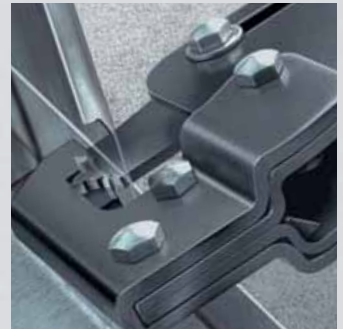
The punching tool is pressed through the metal section sheets
