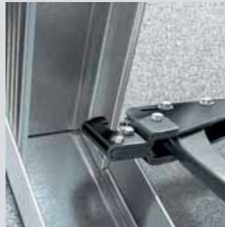
Setting the plier for connection of two metal section sheets
