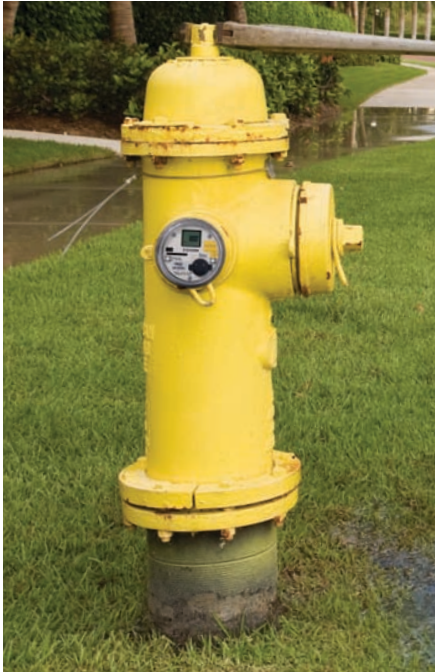
Fire hydrant adapter (A793) necessary to connect to fire hydrants.
